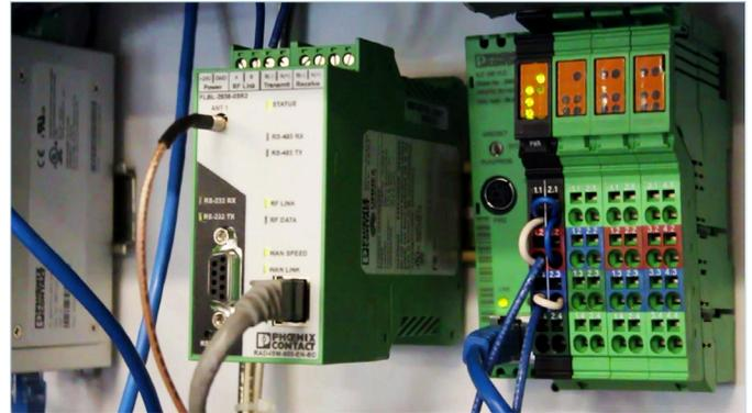
**The ILC controller acts as a communications gateway to the system's legacy PLCs, communicating via EtherNet/IP to Modbus/TCP, then to Modbus RTU via a com server. The TWE radios then transmit this data back to the authority's headquarters.**
