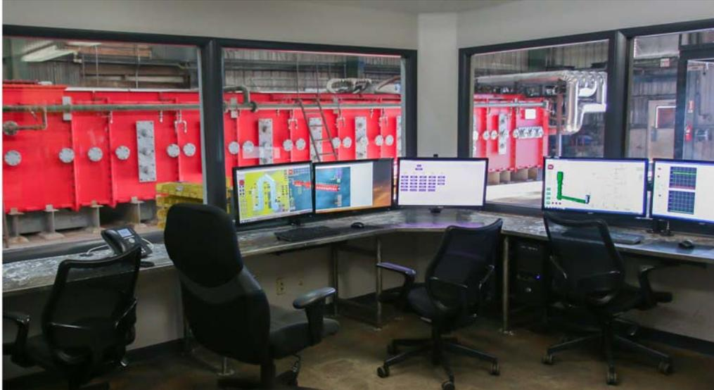
Figure 4: All operations of process equipment at ICGRS can be monitored and controlled from this central control room.
