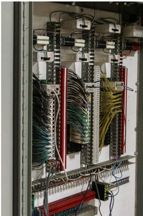
Figure 3: Updating the I/O and controls with modern Opto 22 SNAP PAC hardware was a simple replacement process.
